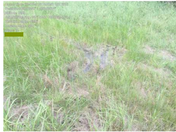
7478 - Exterior Toe (Wet Area)
