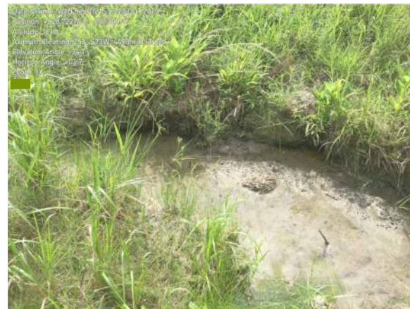
7486 - Exterior Toe (Wet Area)
