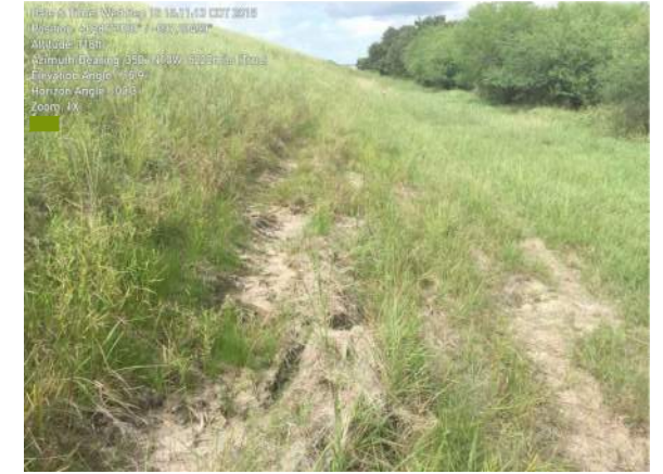
7455 - Exterior Toe (Wet Area)
