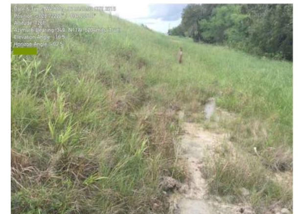
7473 - Exterior Toe (Wet Area)
