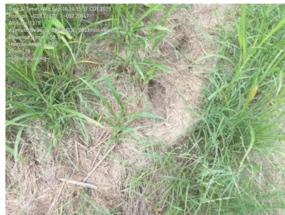
7415 - Exterior Toe (Rodent Grubbing)
