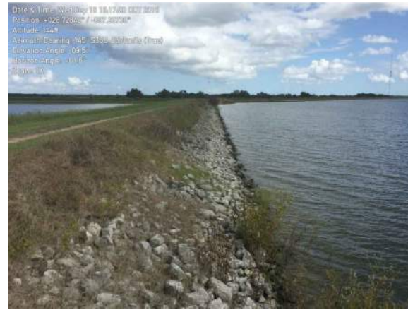
7545 - Interior Slope Protection
